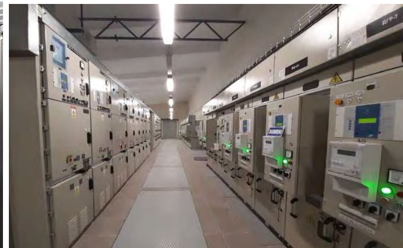
December 2024 – final successful commissioning of GPP1 from Rostekhnadzor
